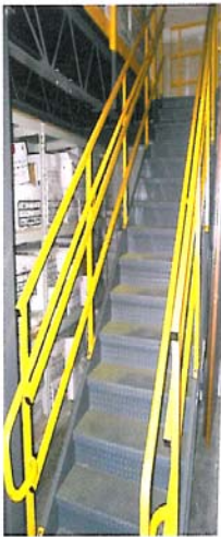
Code-compliant stairs and landings
